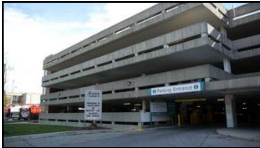
Main Parking Garage on 835 King St. West.
